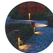
05 Bollard Site Lighting
